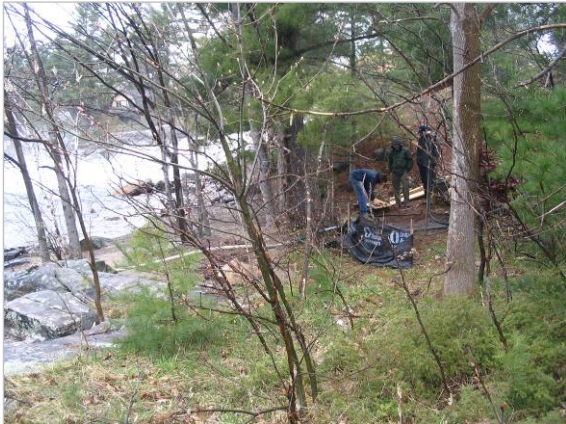
Plate 13: View to northwest showing drilling rig on “dressed and levelled site” of 1924 Bala No. 2 power station.
