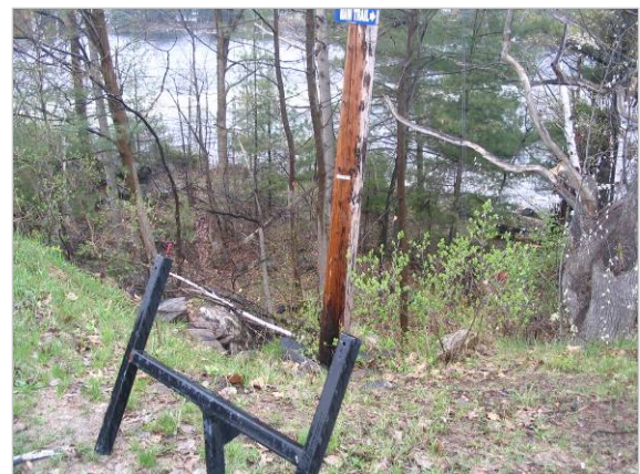
Plate 12: View of proposed power station location. Water intake will pass under highway at this point.
