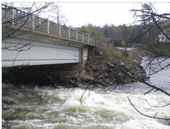
Plate 15: View across channel of South Bala Falls with rock filled road bed covering a granite point extending out from the shore.
