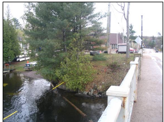
Plate 4: Highway 169 bridge over North Bala Falls channel showing an area of potential near trees on left.
