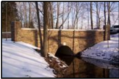
Figure 47 Precast concrete culvert with portal designed as a bridge. Source: Contech Construction Products Inc. www.contech-cpi.com
