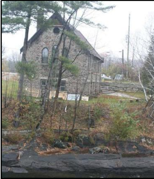
Figure 25 Rear of the former Church facing the South Channel. Stone retaining wall can be seen on the right of the church. The church property appears to have been filled to create a relatively levelling building site.
