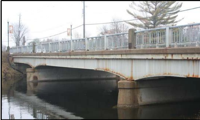
Figure 11 Haunched steel girder structure of Highway 169 over the North Channel.
