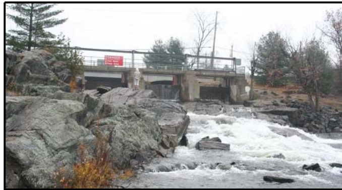
Figure 12 Looking up the North Falls to the 1958 control dam
