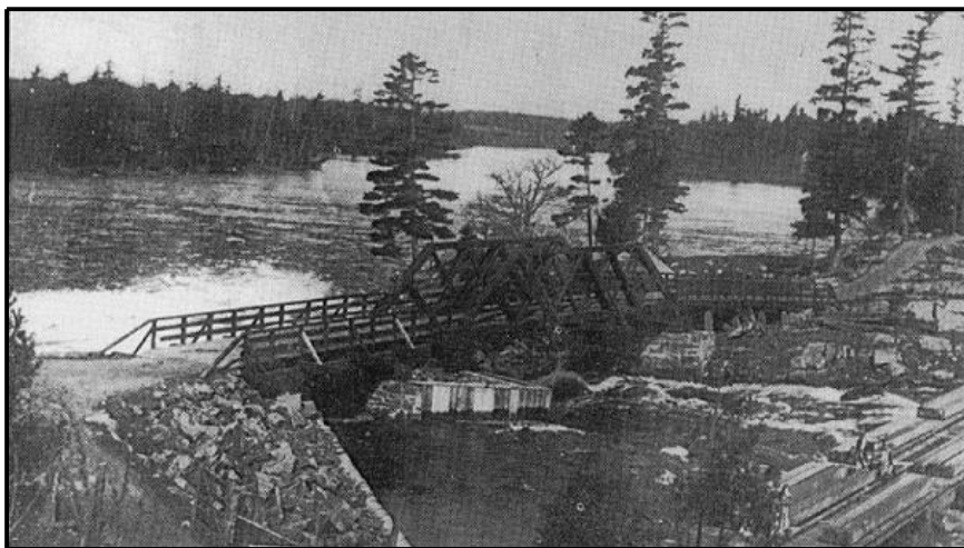
Figure 31 Looking downstream to the 1901 bridge. Stop logs are lying on top of dam at right. Source: Petry, Bala
