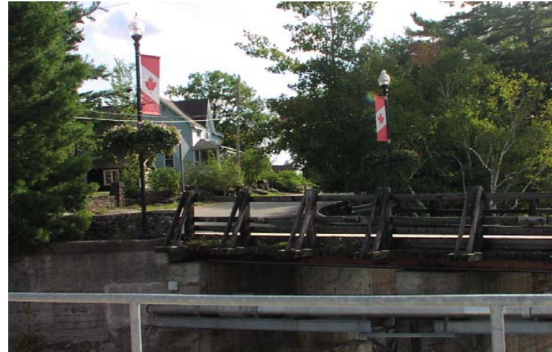
Photograph 4 - Bala Falls Road Bridge
