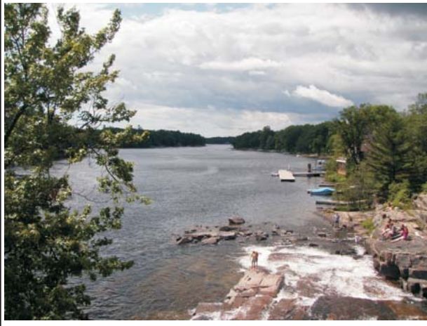
FROM DAM, DOWNSTREAM
