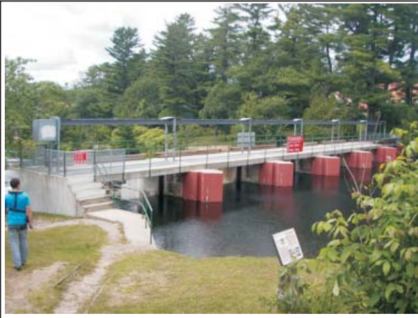
FROM UPSTREAM, DAM SHOWING MESHED GUARDRAIL ENDS AND DANGER SIGNS
