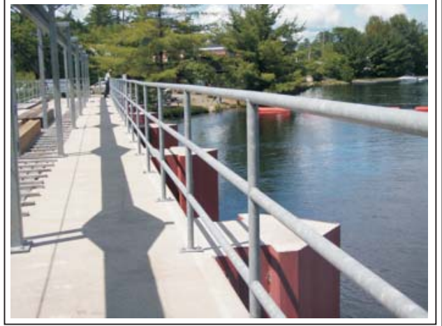
RAILING/BARRIER AROUND DAM DECK
