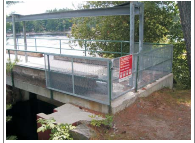
MESHED GUARDRAIL AND DANGER SIGN, NORTH END
