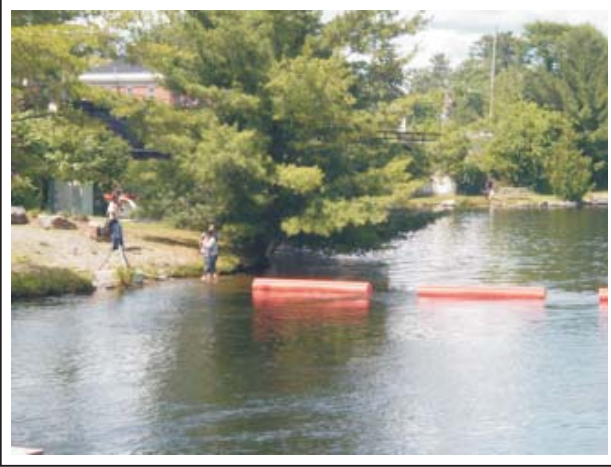
FROM DAM, UPSTREAM NORTH BANK
