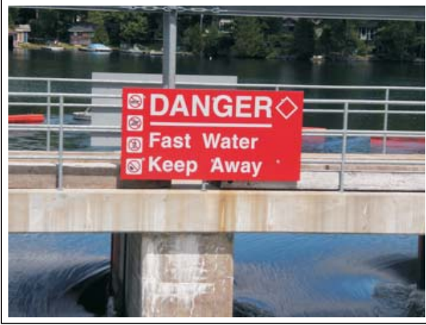
FROM DOWNSTREAM, DAM DANGER SIGN
